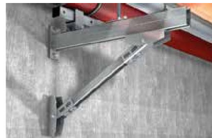
Heavy pipe on shelf
